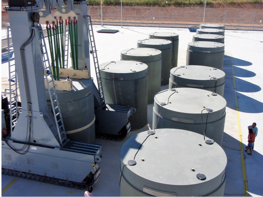
Image of the Individualised Temporary Storage at the José Cabrera nuclear power plant.
